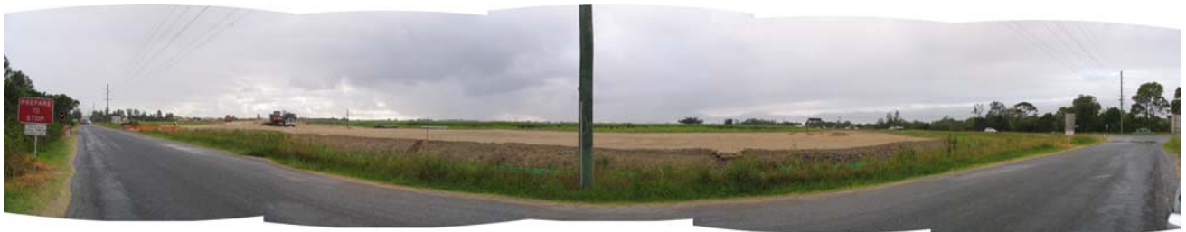
View from Teven Road near its intersection with the Highway looking east – Subject site in middle ground immediately beyond the road works construction.
